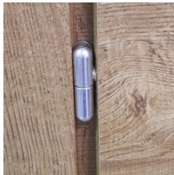
Cerniera Anuba porta chiusa Fiches Anuba porte fermée Anuba hinge with closed door
